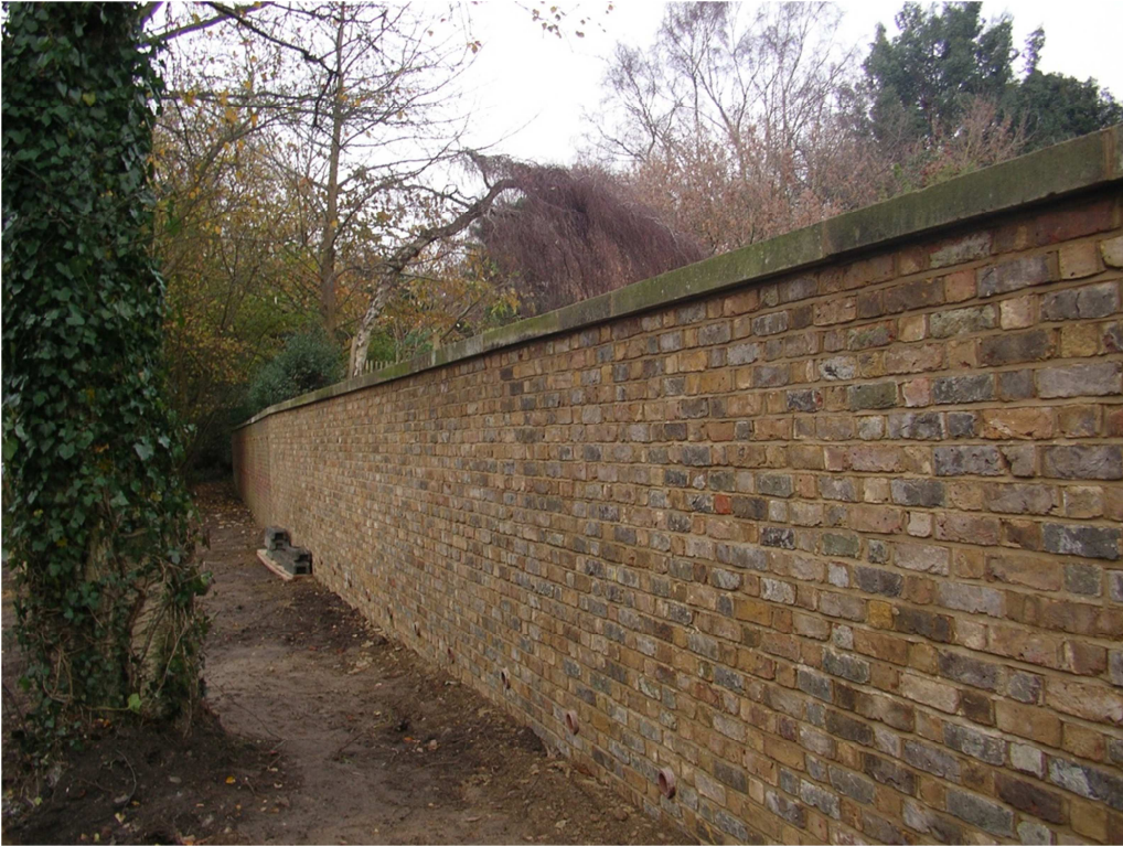
Photograph 7: Completed boundary wall repairs
