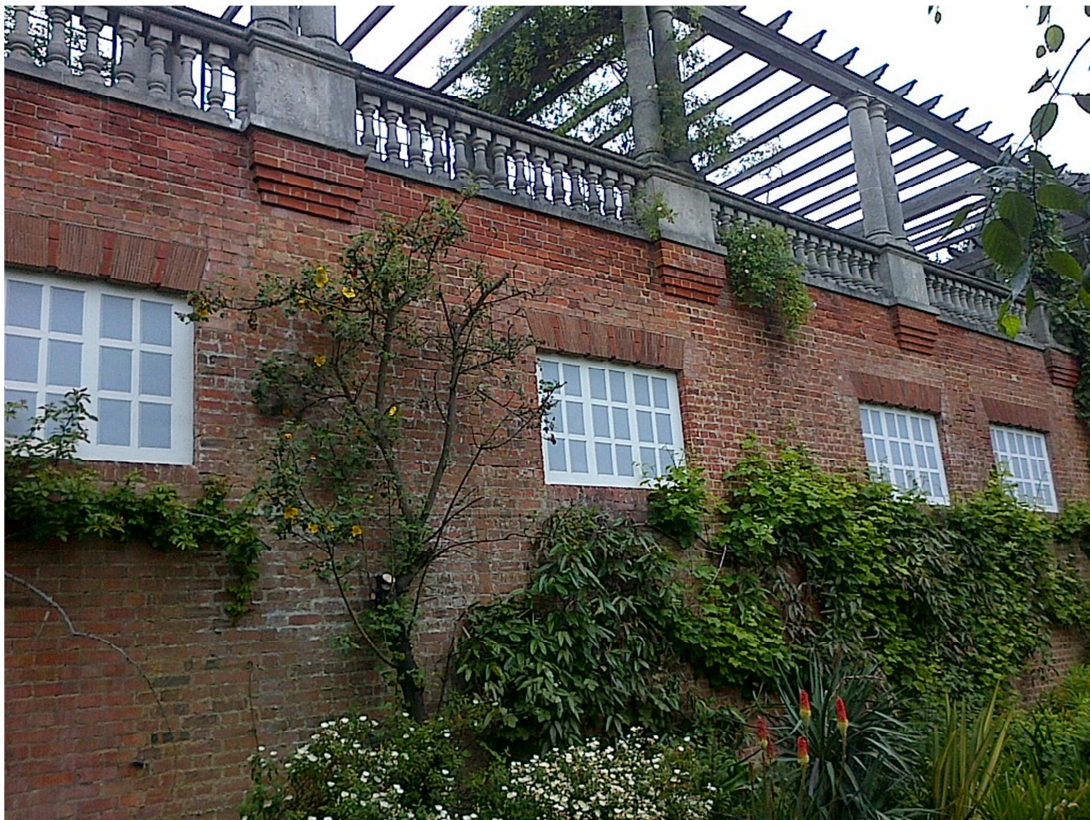
Photograph 3: Re-rendered false windows after works
