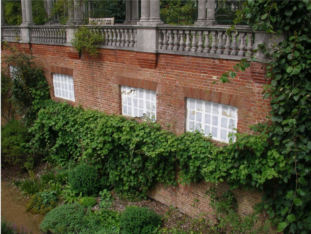
Photograph 2: Re-rendered false windows before works
