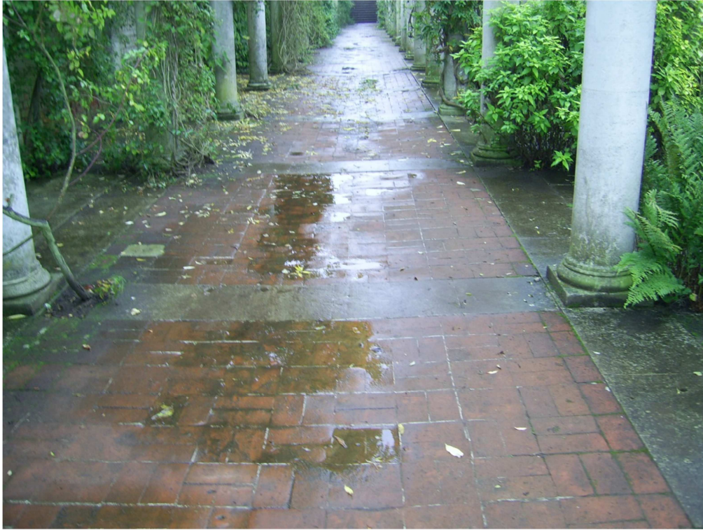
Photograph 4: Paviour pathway before replaying works
